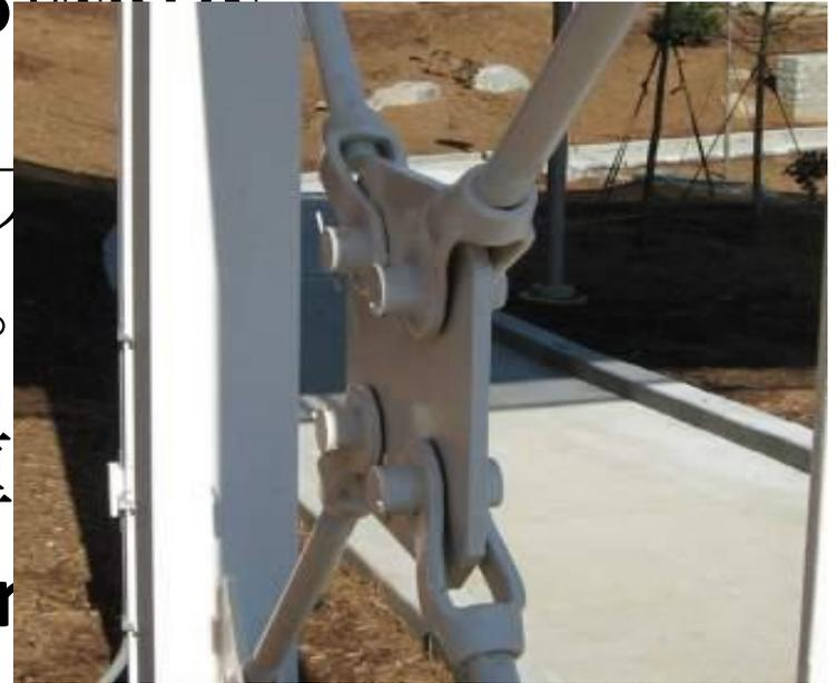
壓緊螺栓，這項接觸應力，稱為**支承應力(bearing stresses)**
